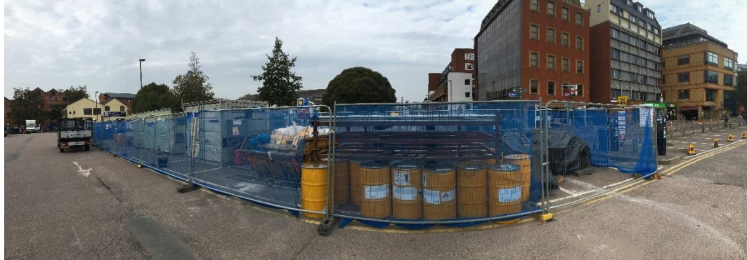
Figure 29. Bedford Road Surface - Works
