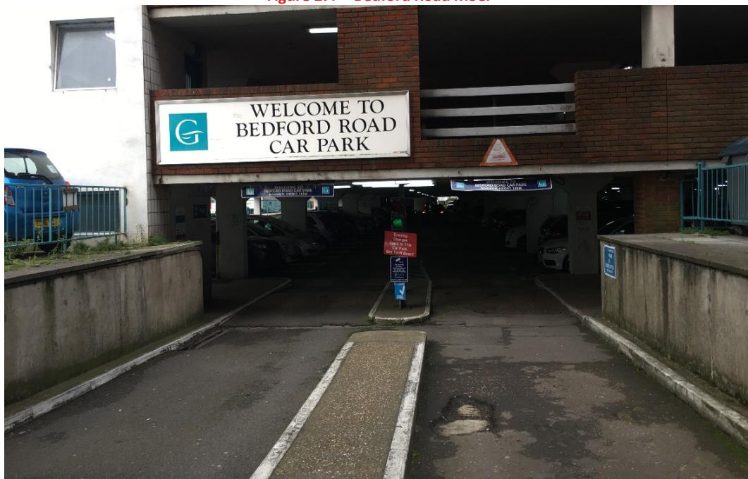
Figure 27. Bedford Road MSCP
