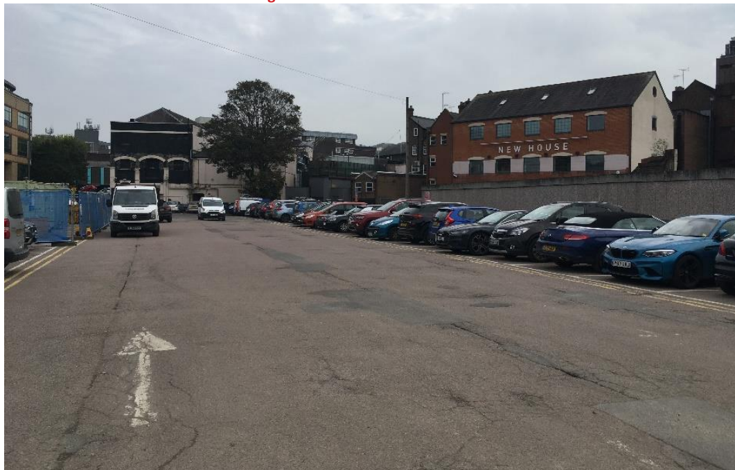
Figure 28. Bedford Road Surface
